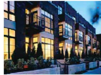
Encroaching Habitable Space (4.5.9)
