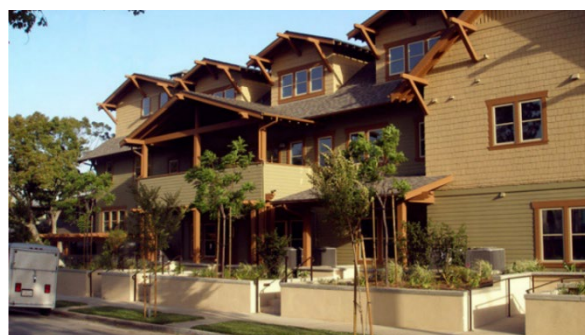
Craftsman Style used for multi-family structure is common throughout the San Gabriel Valley
