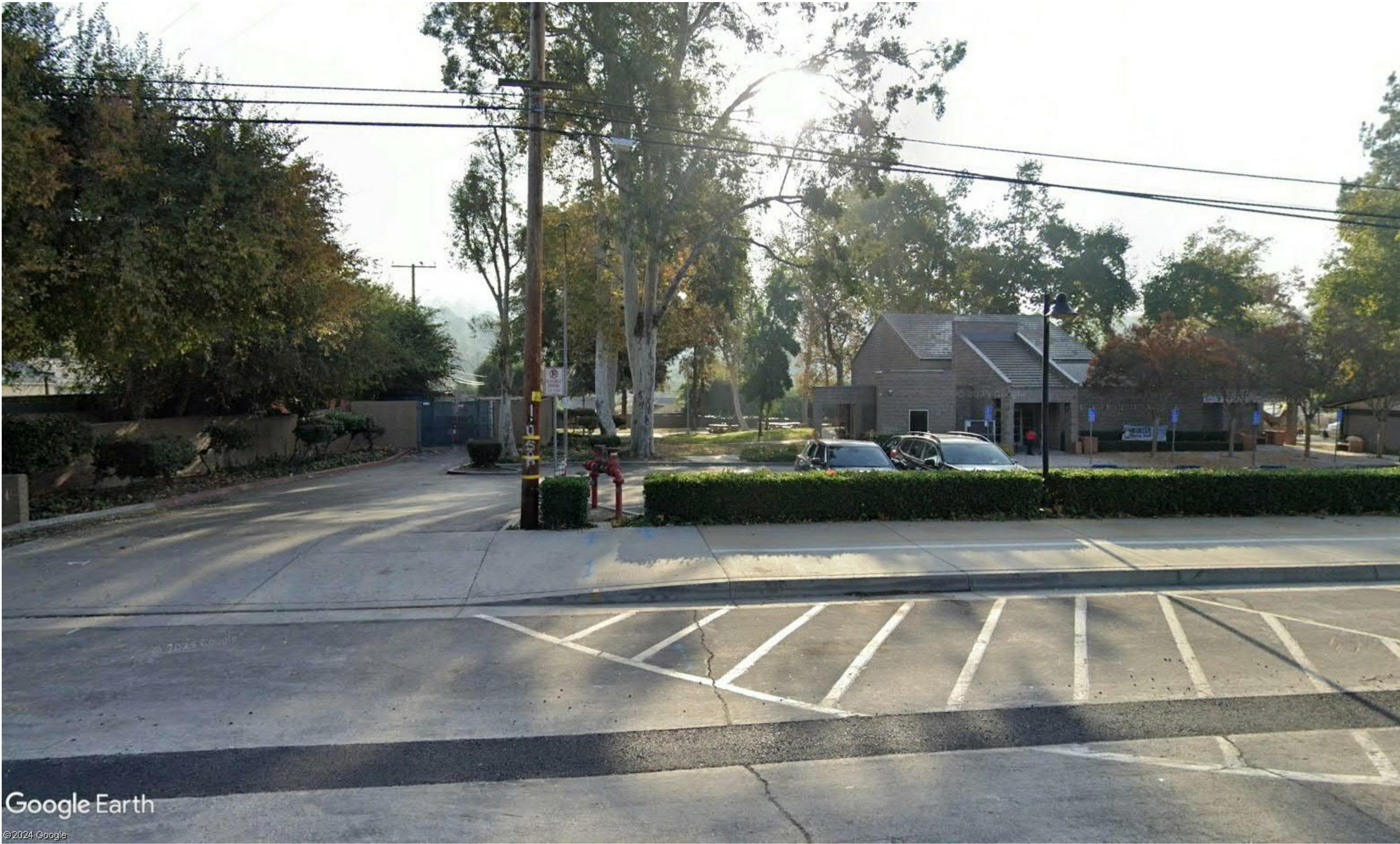
EXISTING BUILDING LACKS STREET PRESENCE
