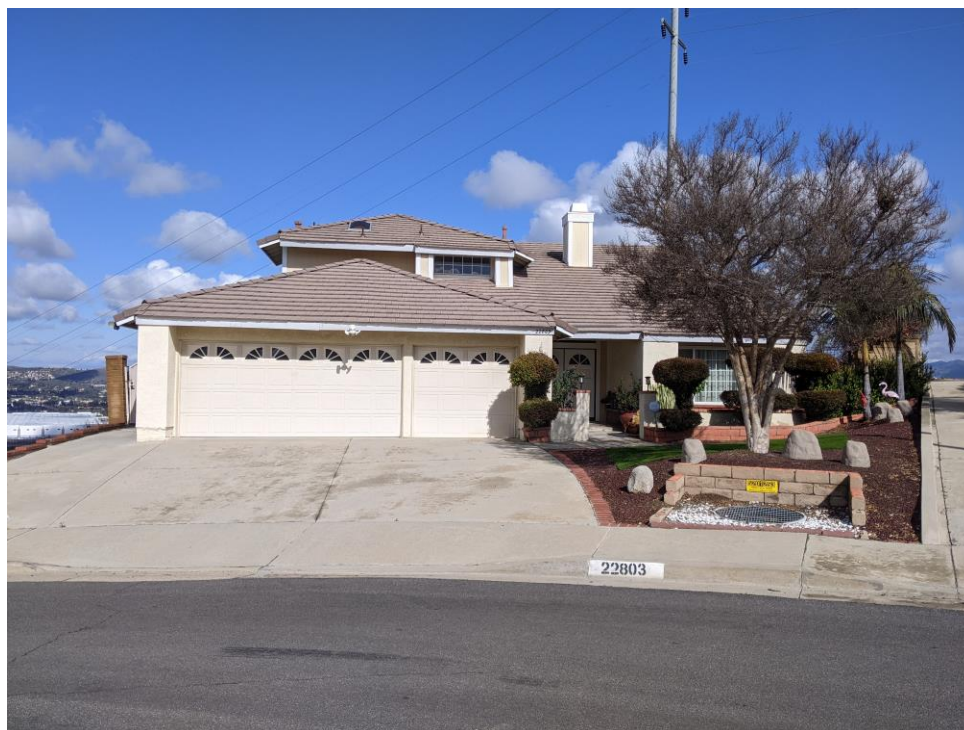
Adjacent Property to the North (22803 Rio Lobos Road)
