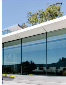
EDW 101 EXTERIOR DOORS AND WINDOWS MANUFACTURER: STYLINE FRAME: PAINTED ALUMINUM COLOR GREY RAL 7016 GLAZING: CLEAR LOW IRON GLASS
