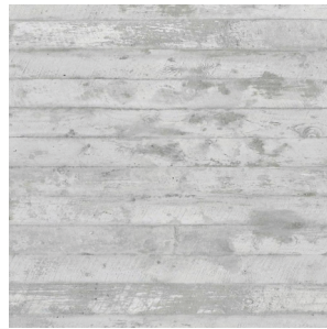
BOF 101 BOARD FORMED CONCRETE WALL FINISH: 4" PINE WOOD BOARD FORMED W/ 1/4" JOINTS COLOR: NATURAL CEMENT COLOR (LIGHT GREY)
