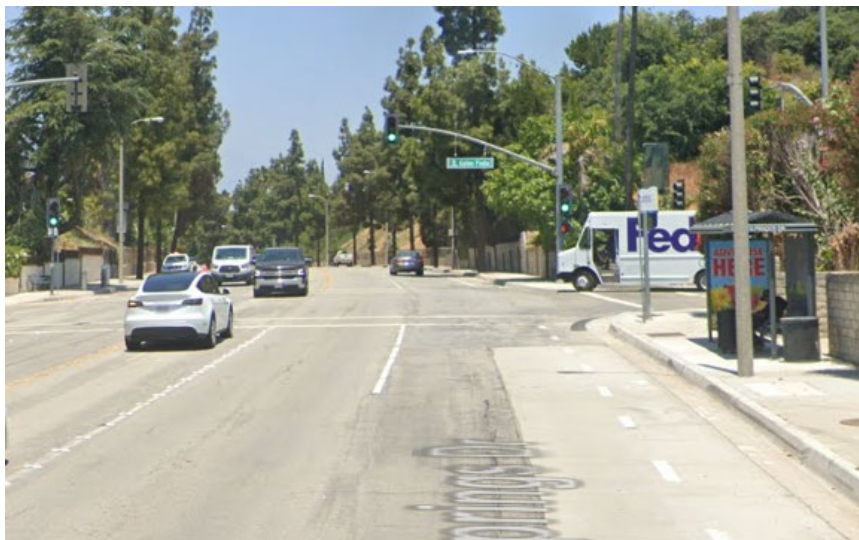
Exhibit 3 – Limited Sight Distance of Northbound Golden Springs Dr for Westbound Golden Prados Dr Vehicles
