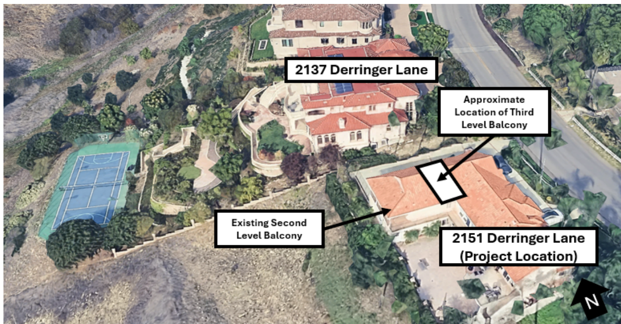
Aerial View of 2137 Derringer Lane from Project Site
