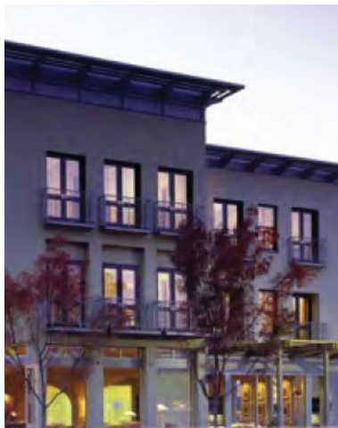
Figure 6-52 - Roof Articulated with Projected Metal Overhang Serving as a Cornice
