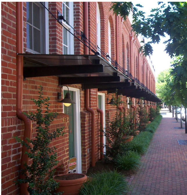
Figure 3-15 - Projecting Canopies Canopies create a rhythm along the streetfront and accentuate the building entrances.
