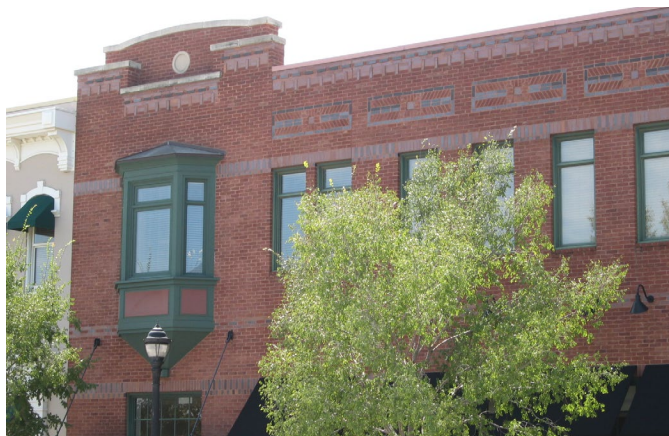
Figure 6-11 - Roof with Detailed Parapet
