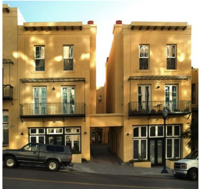
Figure 2-14 - Flex/Loft Building Illustrative Photo
