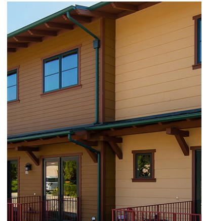
Figure 6-26 - Gutter and Downspout
