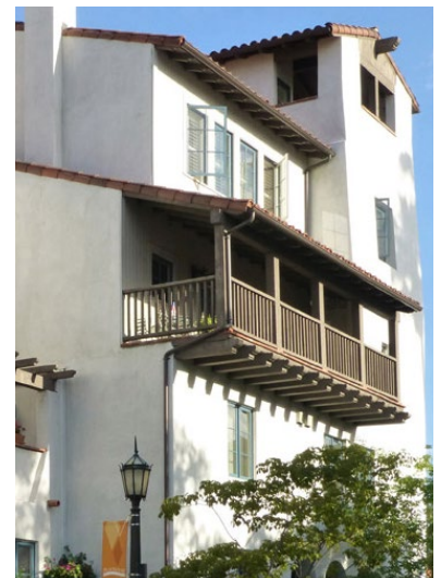
Figure 6-19 - Balcony Overextending Sidewalk
