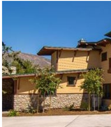
Figure 6-25 - Masonry and Stone Base
