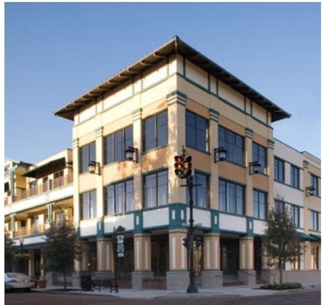
Figure 2-29 - Wrap Building Illustrative Photo Street view of a linear building. The Façade does not reveal the parking use behind.
