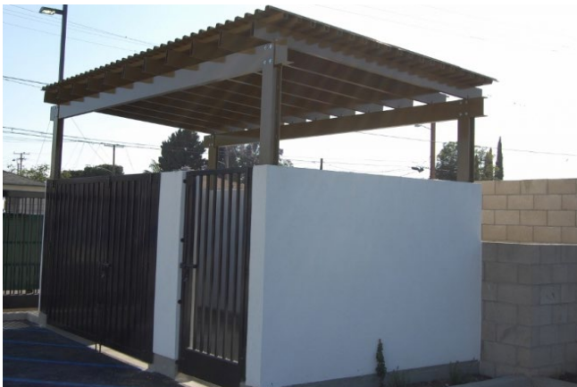
Figure 5-8 - Service and Auxiliary Equipment Illustrative Photo
