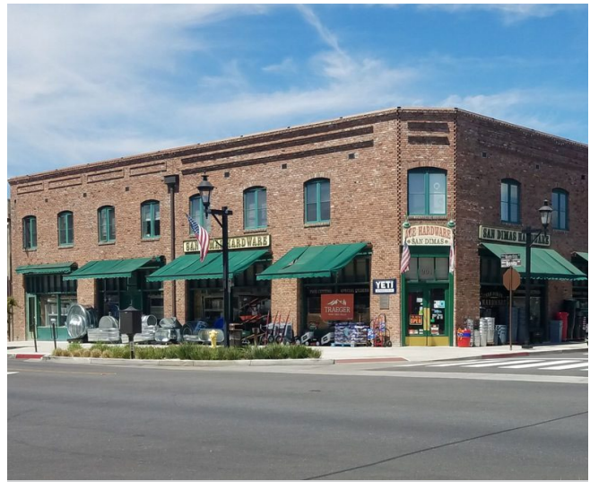
Figure 2-25 - Small Mixed-Use Building Illustrative Photo
