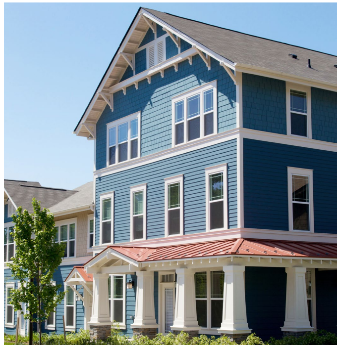
Figure 6-32 - Bracketing of a Roof Gable
