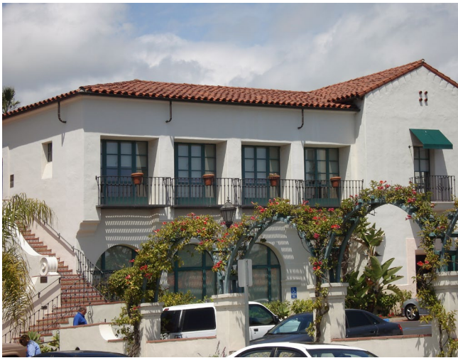
Figure 3-12 - Windows Windows are recessed from the exterior wall surface.
