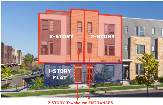
Figure 2-7 - Illustration of a Townhouse Stacked over a Separate Flat
