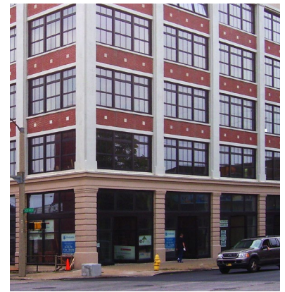
Figure 6-4 - Large Windows Ground Floor
