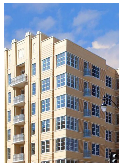
Figure 6-41 - Undulating Parapet
