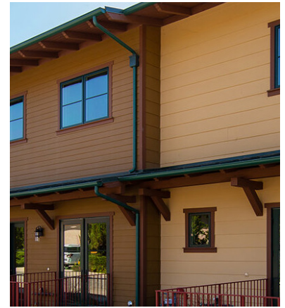
Figure 6-26 - Gutter and Downspout
