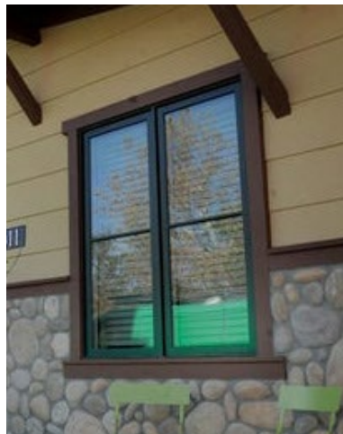
Figure 6-27 - Paired Openings Composed Horizontally
