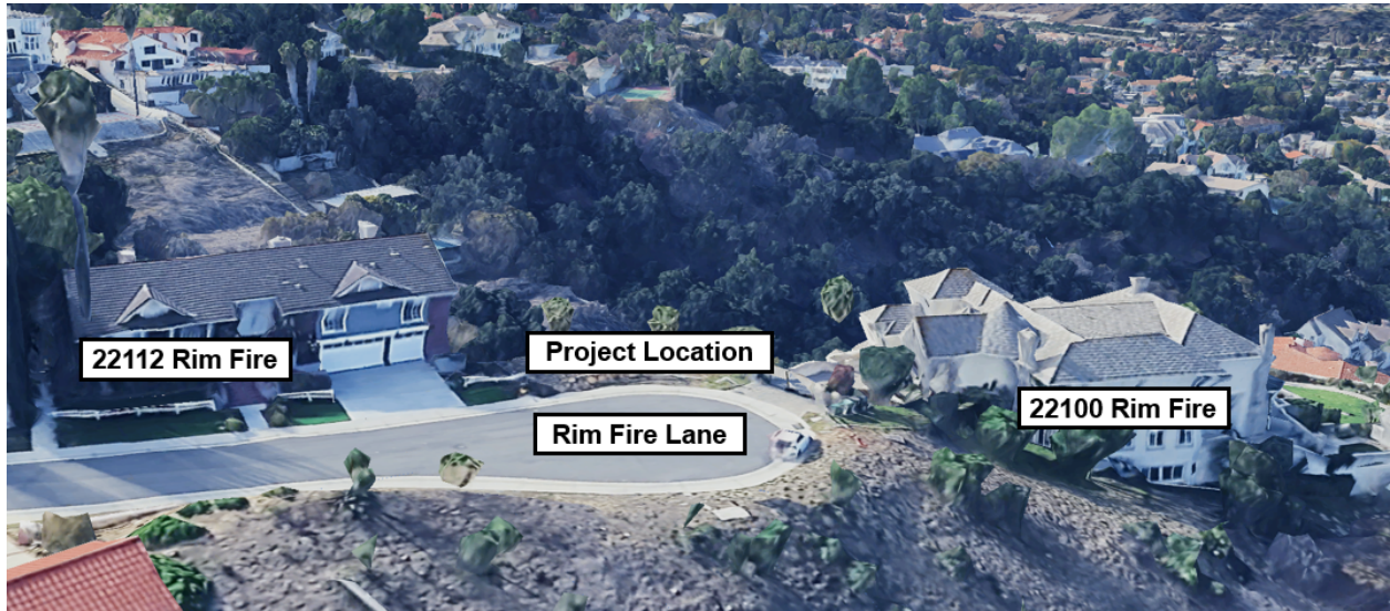
Aerial View of Project Site and Adjacent Properties
