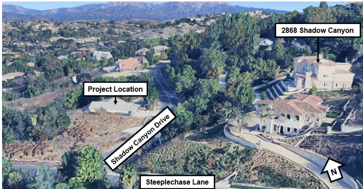
Aerial View of Project Site and Adjacent Properties
