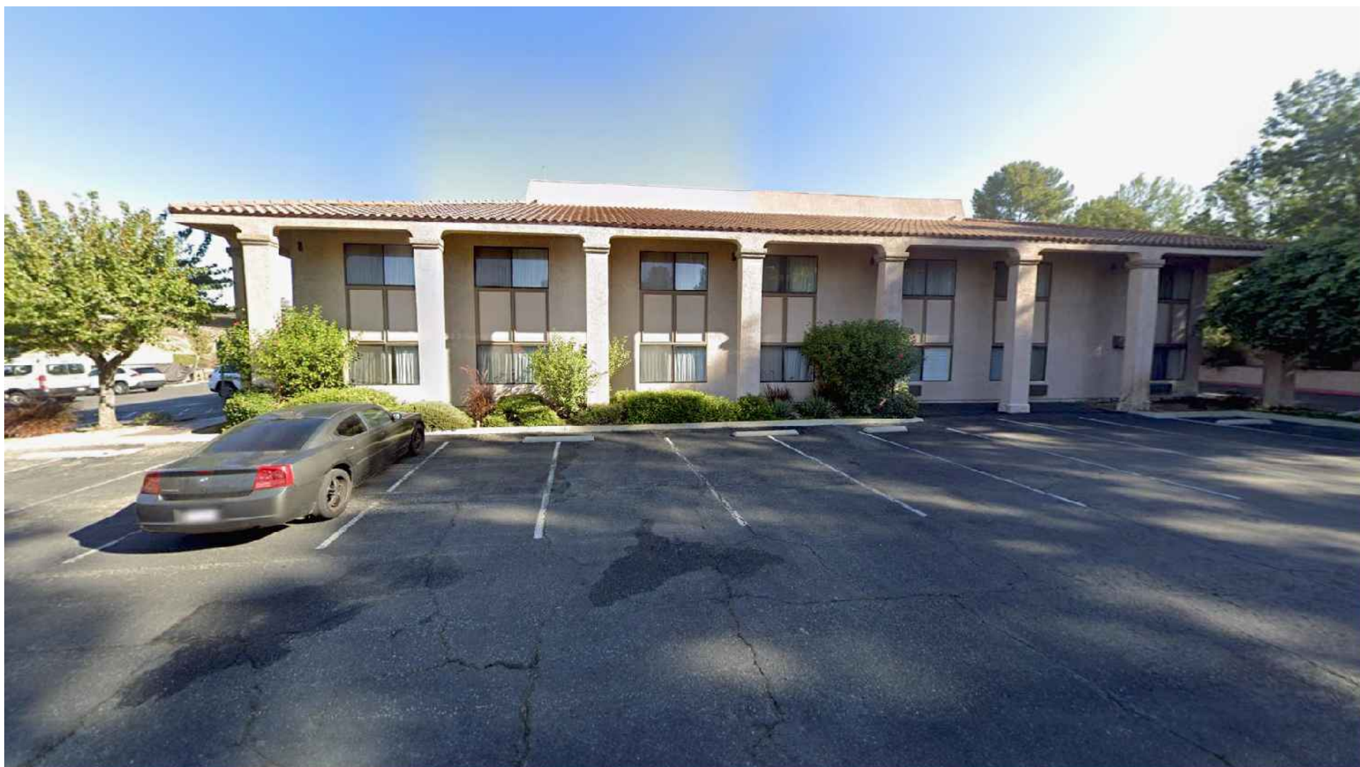
5 NORTH VIEW FROM SITE FACING BEST WESTERN HOTEL
