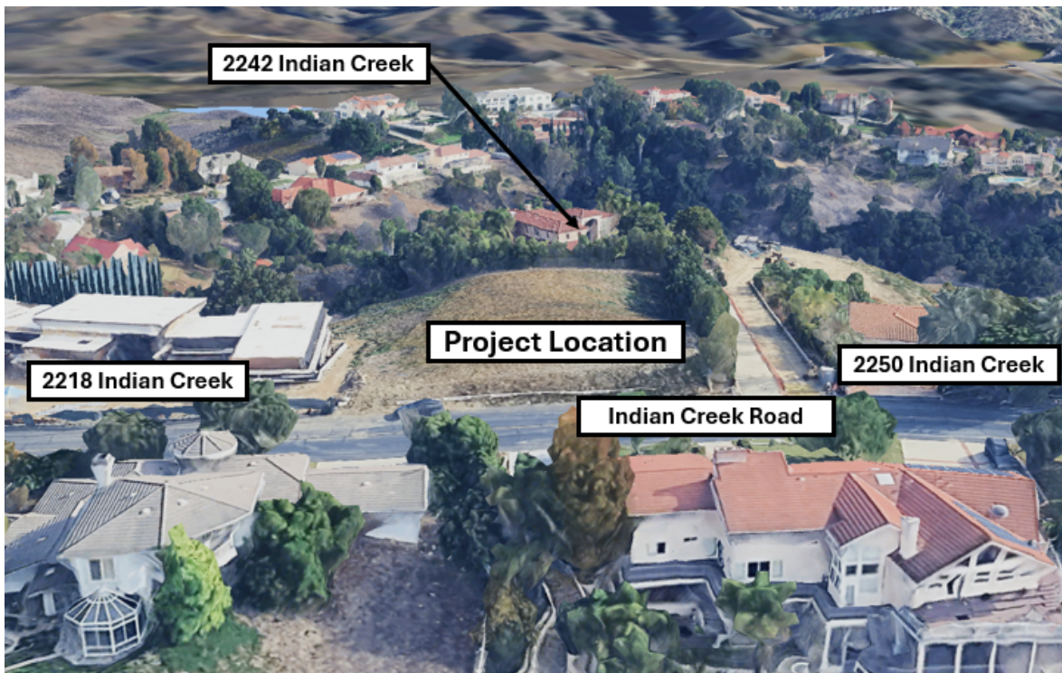
Aerial View of Project Site and Adjacent Properties
